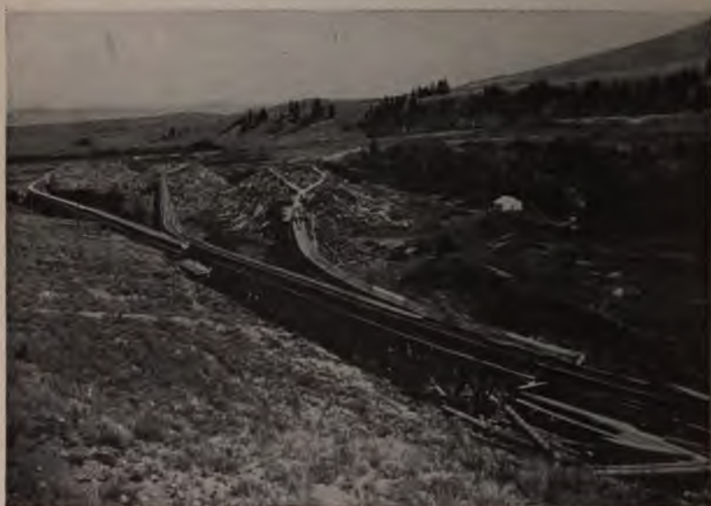
FIG. 127.—The Terminal of a Log Flume, near the Deerlodge National Forest, Montana. This type is known as an "elephant."
